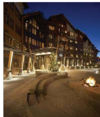
One Steamboat Place skirts the perimeter of the base village and is a gateway to the revitalized Gondola Square
