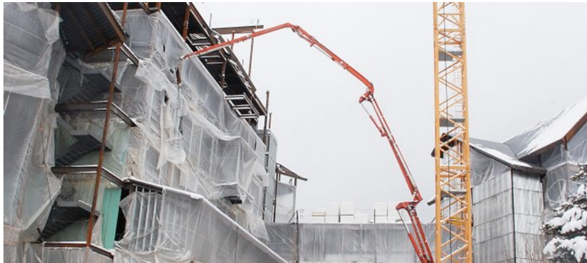
More than 300 construction workers bustle through the One Steamboat Place site daily. Construction is said to be on schedule for completion late in 2009. Enlarge photo — Photo by Tom Ross
